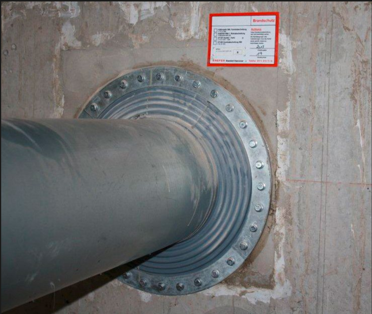
Fire protection bulkhead of type W200FS + W410FS for large pipe movements between machines house and boiler house
